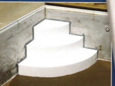
Ready for the liner... Total time 30 minutes!
