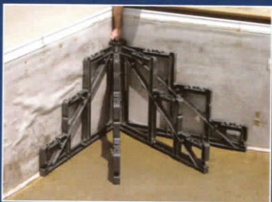
Erect bench supports on solid base
