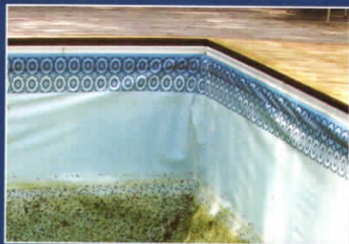
Remove old liner
