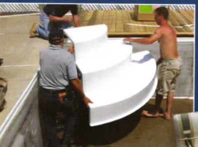
Cover with preformed shell
